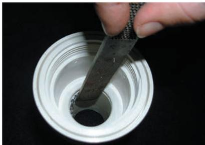
If hole is blocked with glue or pipe shavings use a file or knife to trim until the Pool Valet Retro nozzle will fit into the pipe.
